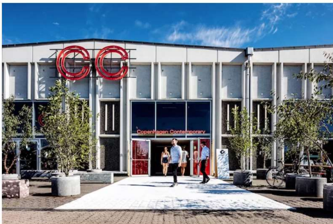
Entrance to Copenhagen Contemporary. Photo: Anders Sune Berg
